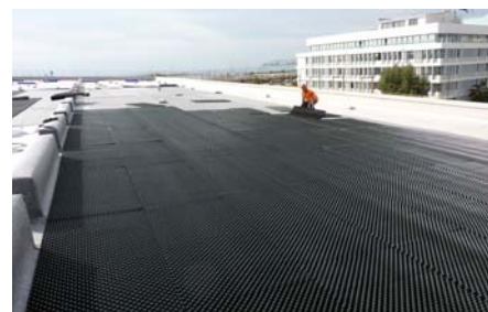
The Floradrain® FD 40-E elements below the vegetated areas allow for a quick runoff of exceeding water.
