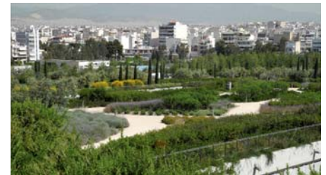
Protectodrain® PD 250 was applied as a base for the walkways over the car park. © HPA
