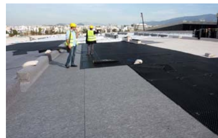
The Protection Mat ISM 50 was laid over the multi-layer waterproofing.
