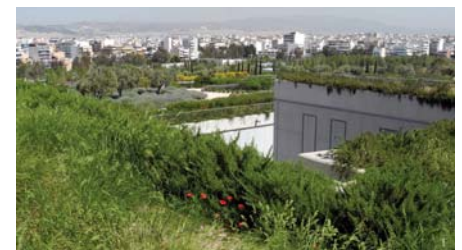
A look between the opera and the library over the car park shows the diversified design. © HPA
